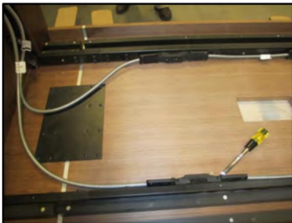
Step (2): Join the two sides of the table together with a connector receptacle
